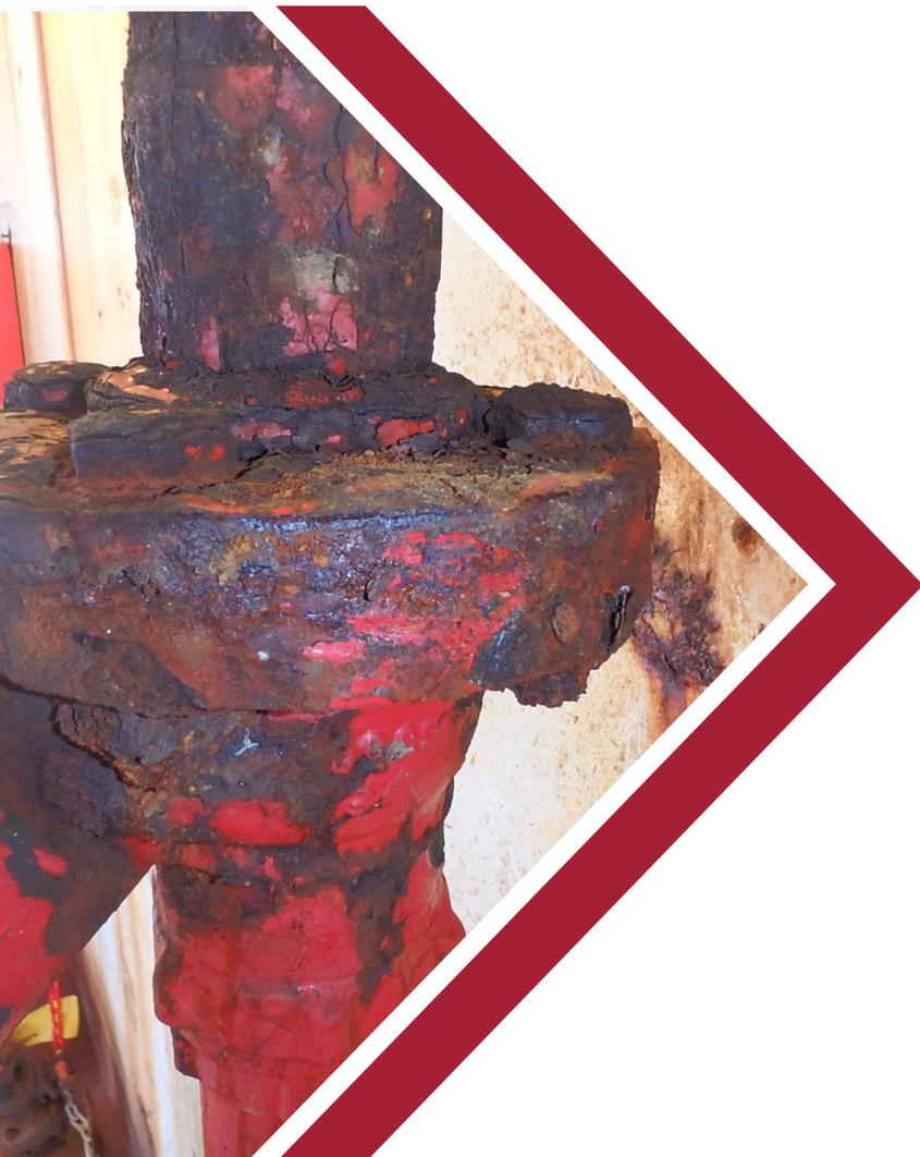
**Corroded bolted flanged joints are widespread on the UKCS and establishing their condition and ongoing integrity is important for safe and reliable operations.**
